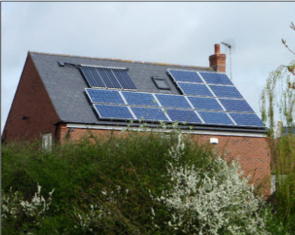
A local 3kW installation showing several Solar PV (electricity-generating) modules and, top left, a Solar Thermal (hot water) panel.
